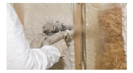
Spray Polyurethane Foam (SPF) is an insulation product that is produced on-site and is typically applied by certified applicators. Two liquid components, polymeric MDI (A) and a polyol blend (B) are mixed at high or low pressure using a spray gun, and the reacting mix is sprayed onto the substrate. It expands and solidifies to form a polyurethane foam that adheres well to the area it is applied to, providing a seamless seal.
