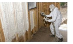
Spray Polyurethane Foam (SPF) is an insulation product that is spray-applied in situ at a building site. Two liquid components, MDI (A) and polyol blend (B) are mixed under pressure and sprayed onto a roof or wall cavity. The reacting liquids expand and solidify into a foam matrix creating a seamless seal. SPF adheres well to the area it is applied to, providing an air barrier that prevents thermal leaks.
